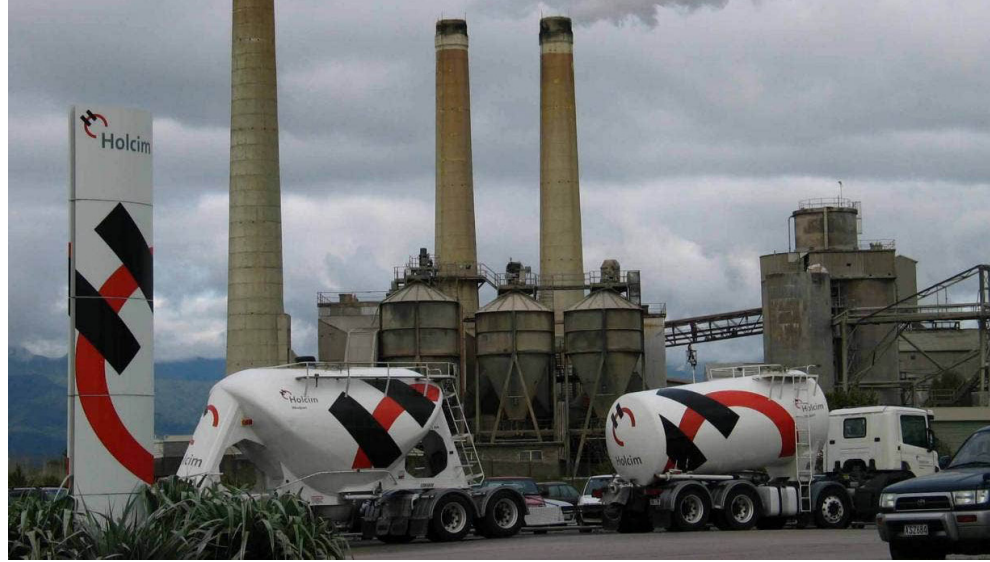
Holcim's New Zealand cement plant.
